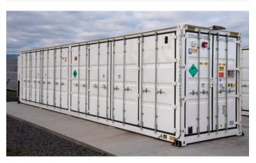
By locating battery cells in specially designed enclosures equipped with advanced safety and fire suppression systems, today's BESS systems greatly diminish the likelihood that any singular battery cell failure will cascade into a larger thermal runaway event or fire.
