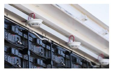
New BESS systems, including the design for Seguro Storage, feature layered active and passive safety, monitoring and fire suppression systems, including flammable gas detection, fire detection and alarm, direct injection fire suppressant and exhaust/deflagration ventilation.
